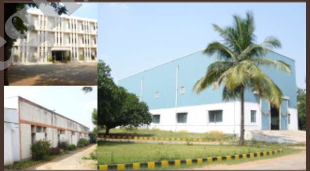
Hydraulic Cylinders & Marine Systems Plant
